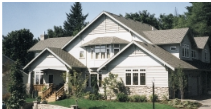
FIGURE 20.14 ■ A gable roof is composed of two intersecting planes that form a peak (the ridge) between the planes.
