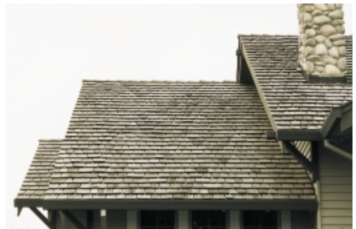
FIGURE 20.36 ■ Cedar shakes are a rustic but elegant roofing material. Courtesy Tim Taylor.
