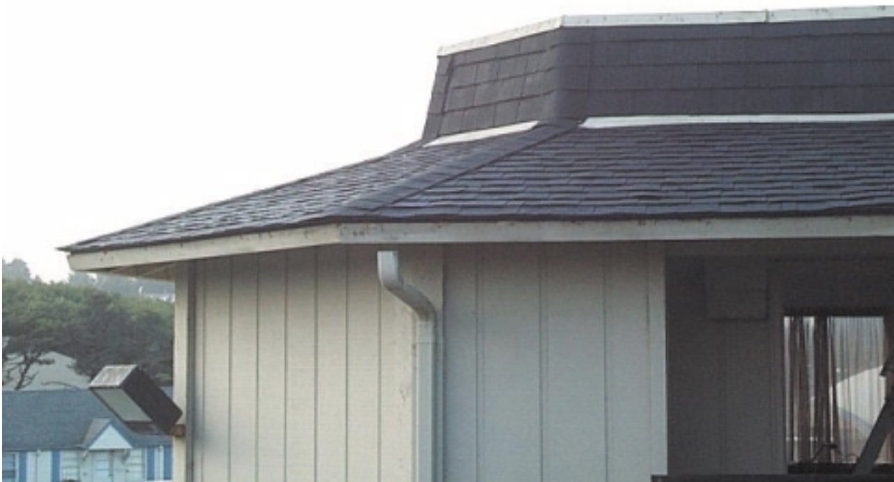
FIGURE 20.28 ■ Mansard roofs are used to help disguise the height of a structure.
