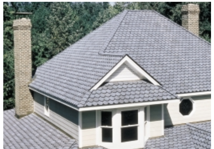
FIGURE 20.25 ■ A Dutch hip is a combination of a hip and a gable roof. Courtesy CertainTeed Roofing.
