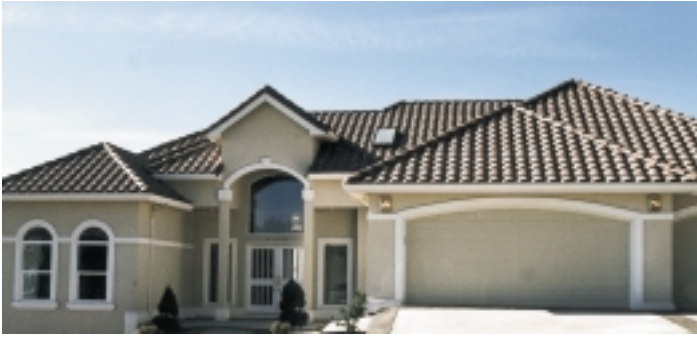
FIGURE 20.23 ■ A hip roof is made of three or more intersecting planes. This home uses a combination of hip roofs with a gable roof over the entry area to create a pleasing roof structure. Courtesy LeRoy Cook.
