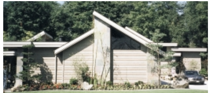
FIGURE 20.11 ■ Many contemporary homes combine flat and shed roofs to create a pleasing design. Courtesy LeRoy Cook.
