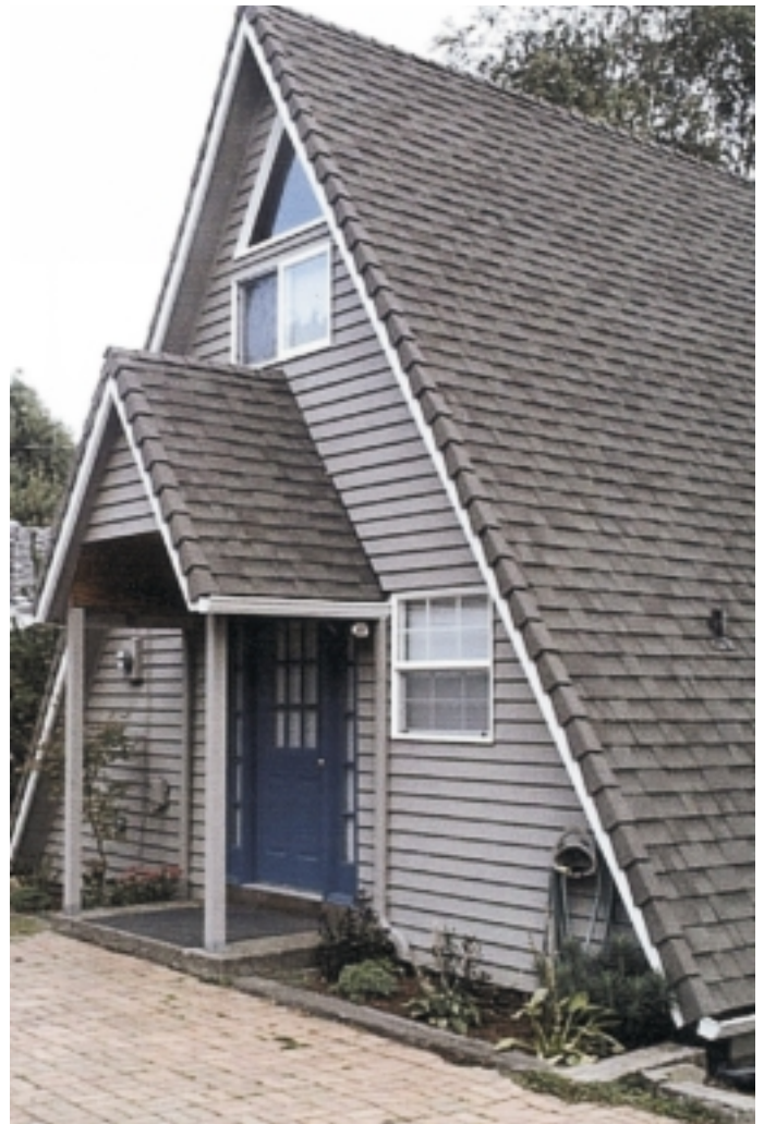
FIGURE 20.17 ■ An A-frame uses a steep roof to form the walls of the upper level. Courtesy Janice Jefferis.
