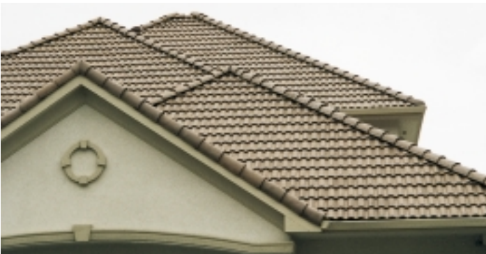
FIGURE 20.37 ■ (a) Tile is an excellent choice for a roofing material because of its durability. Courtesy Tim Taylor. (b) Many tile patterns are made to simulate Spanish clay tiles. Courtesy Tim Taylor.
