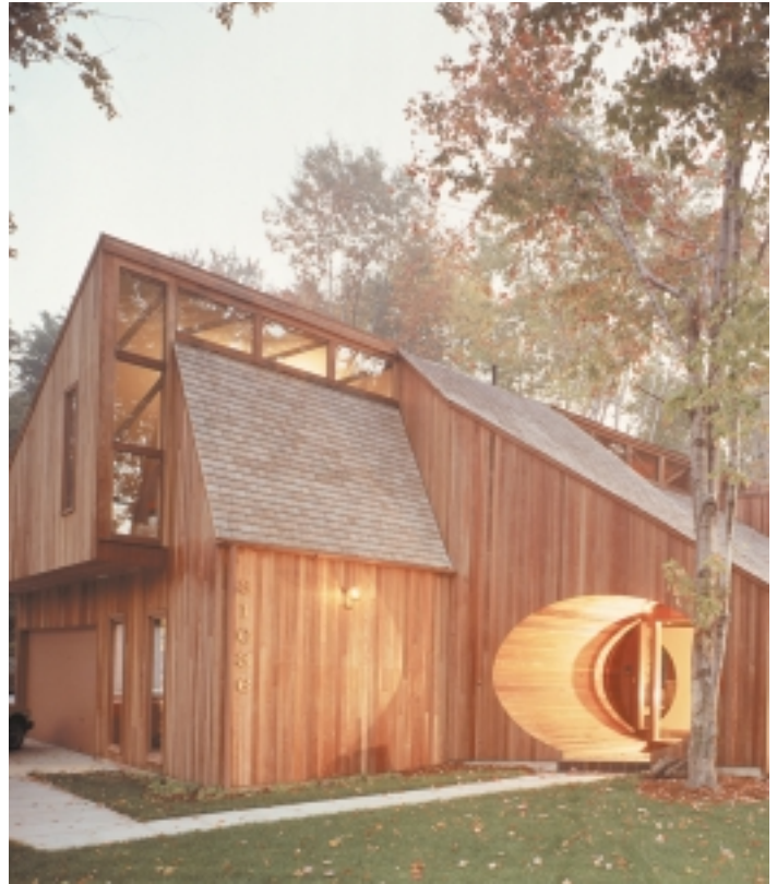
FIGURE 20.2 ■ In addition to aesthetic considerations, the roof is often used to resist wind and seismic forces when walls of the structure contain large amounts of glass. Courtesy of the California Redwood Association, Robert Corna architect, photo by Balthazar Korab.
