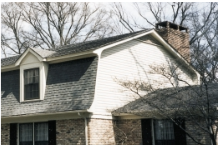
FIGURE 20.20 ■ The gambrel roof is often used to enhance the traditional appearance of a residence. Courtesy Michael Jefferis.
