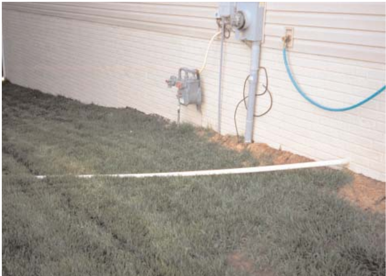
1-23 Exterior portion of sump pump discharge
