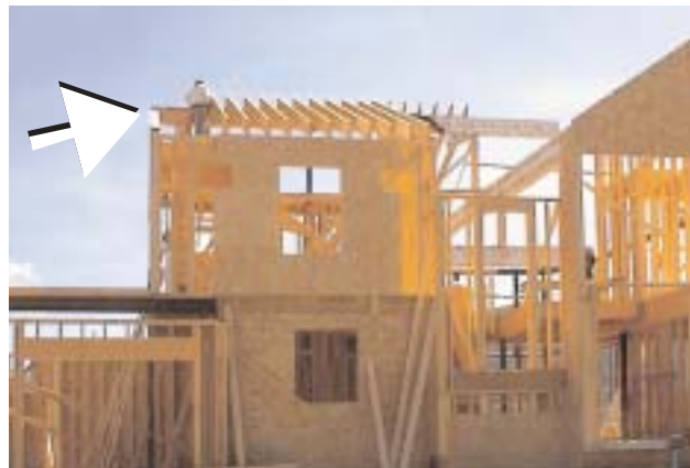
1-18 Joist and rafter roof structure
