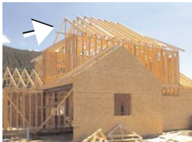
1-19 Pre-fabricated roof trusses in use
