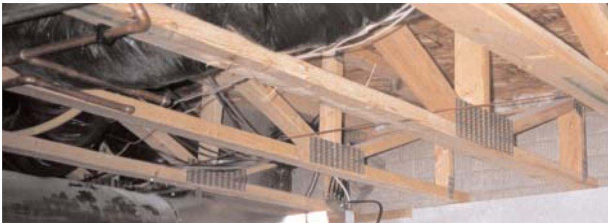
1-13 The underside of a floor built on fabricated floor trusses
