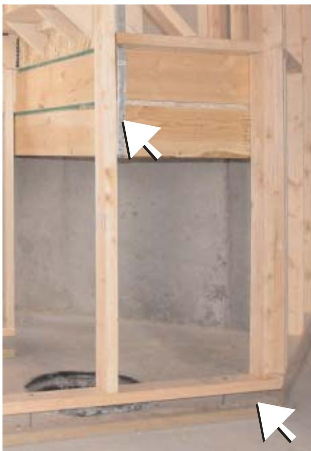
1-14a Floating wall hung from the floor above (note support strap and gap at bottom)
