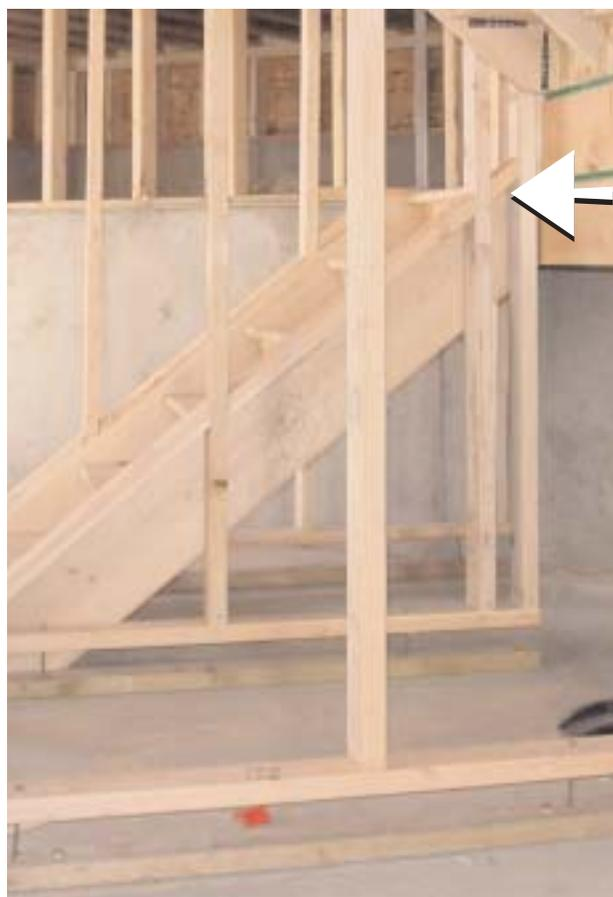
1-14b Hinging at the landing above (arrow) allows the staircase to adjust if the basement floor rises
