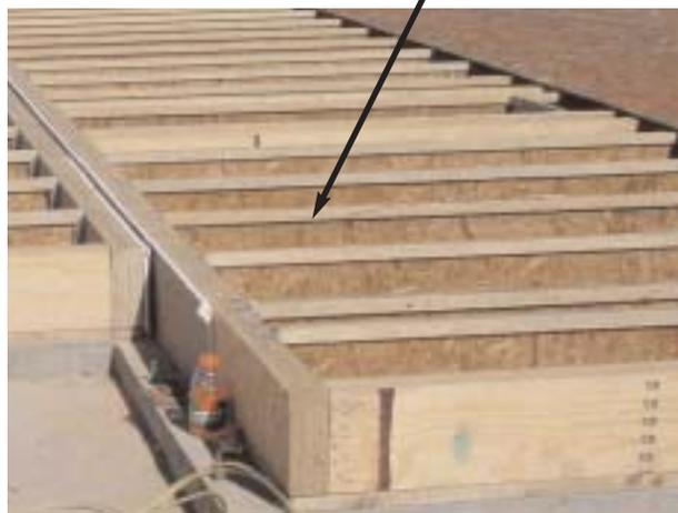
1-12 Framed wood floor system, using I-joists
