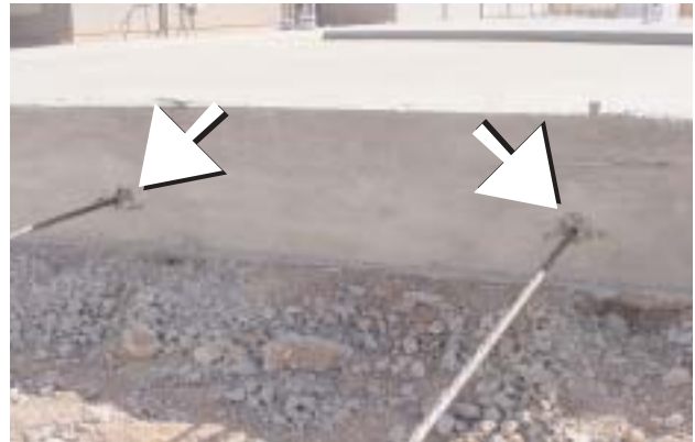
1-06 Slab on grade with tensioning cables
