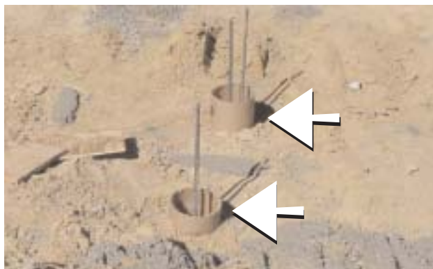
1-04 Caissons shortly after being poured
