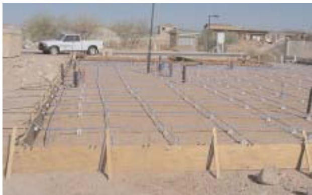
1-07 Form work and tensioning cables ready for concrete pour
