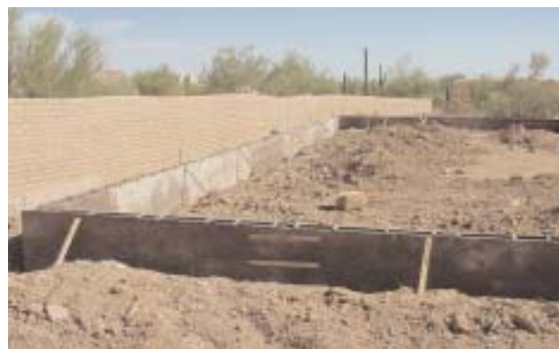
1-11 Perimeter wall with the slab independent of the foundation
