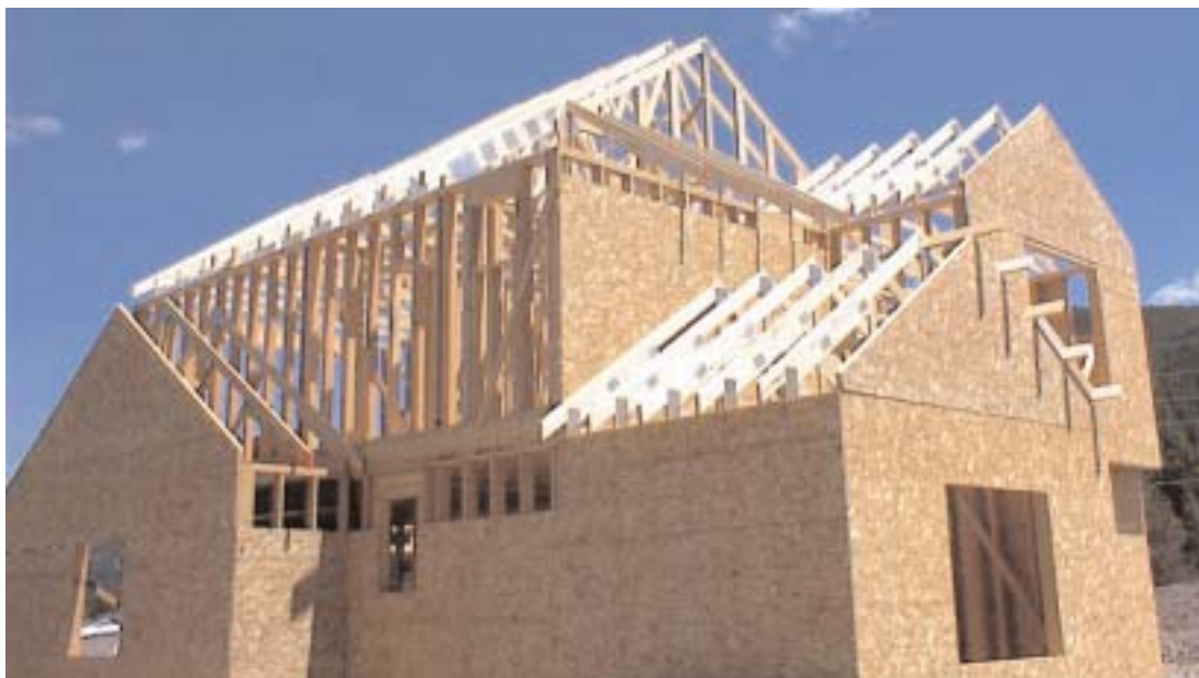
1-01 Load bearing walls supporting the roof
