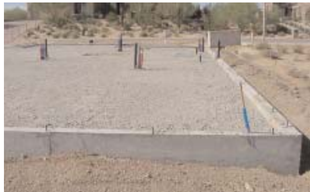
1-09 A slab foundation, after it has been formed and poured
