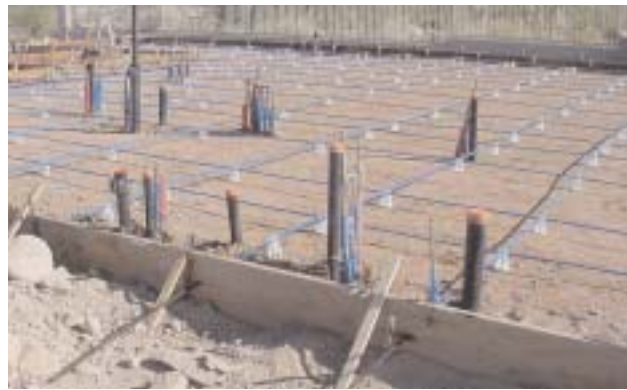
1-08 Form work set up for a poured-in-place foundation
