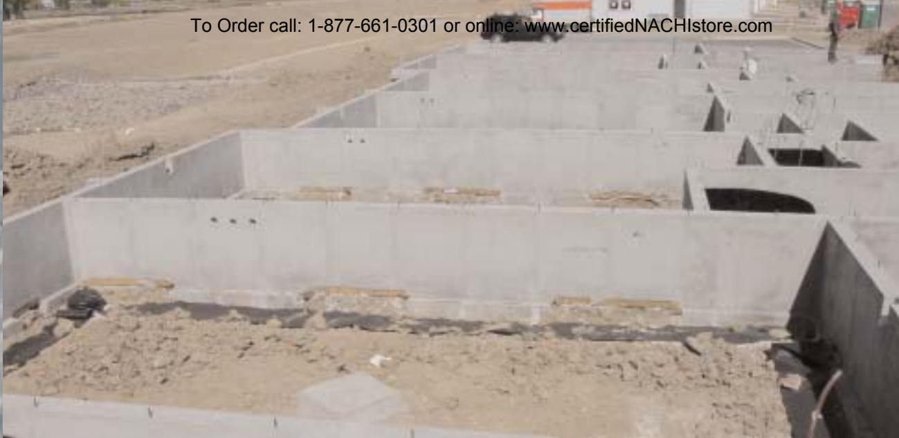
1-03 A grade beam on caisson foundation
